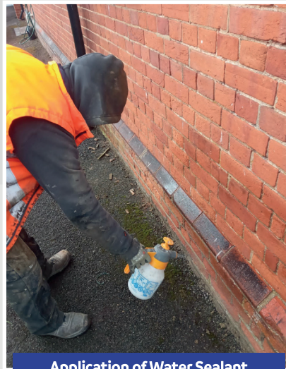
Application of Water Sealant
